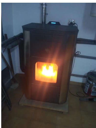
Installation of a pellet boiler in a home. The pictures from left to right: the boiler in operation, the storage of the pellets in the boiler and the pellet bags.
